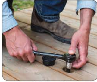
Level any deck from the top with the simple turn of a ratchet.
